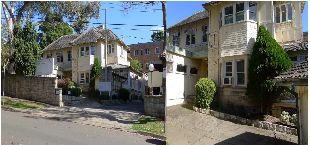
Figure 5: Property Photos (Source: Clive Lucas, Stapleton and Partners Report June 2014)
