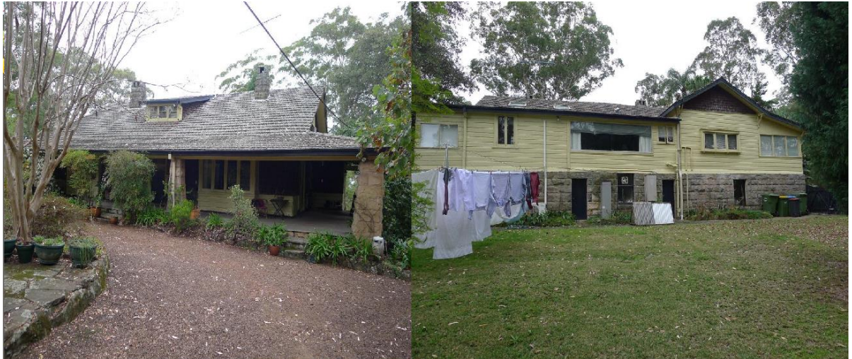
Figure 8: Property Photos (Source: Clive Lucas, Stapleton and Partners Report June 2014)
