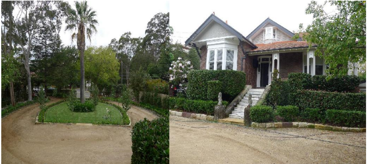
Figure 11: Property Photos (Source: Clive Lucas, Stapleton and Partners Report June 2014)
